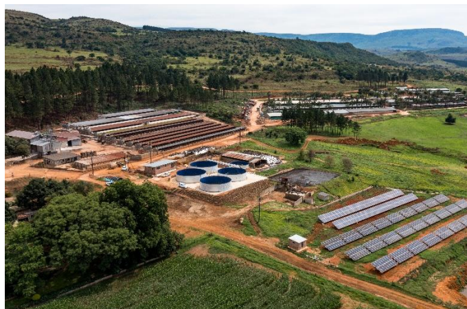
Figure 2: An aerial view of Thiele Holdings, showing the location of the biogas digesters
