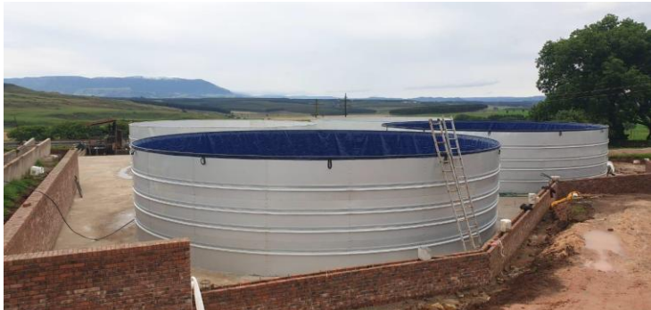
Figure 3: Digesters being installed
